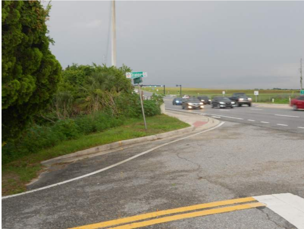
Figure 25: Looking W along S.R. 50 ROW from NW corner
