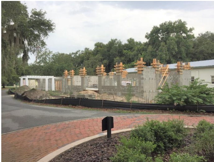
Arts and Heritage Center under construction.
