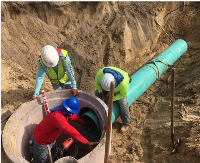
Sanitary Sewer Project - Phase 1C, a.k.a. 'Gravity-One'
