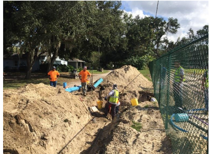
Water Main Construction
