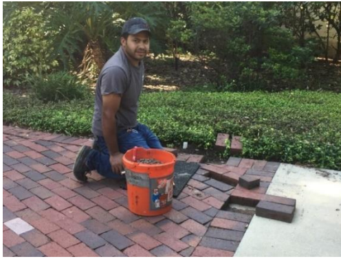
Public Works employee, Luis Reyes, maintaining the Town's brick paver sidewalks.
