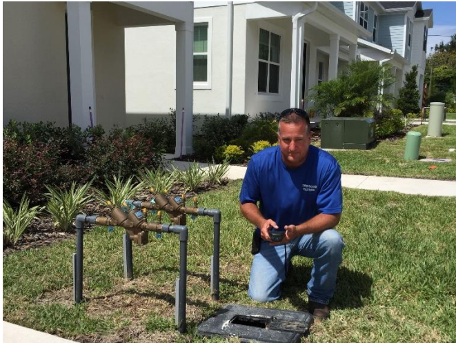
Public Works employee Mike Adams installing a new water meter.
