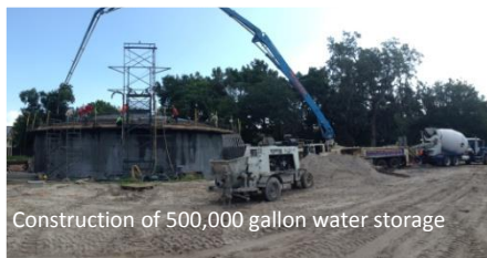
New 500,000 gal tank and distribution house
